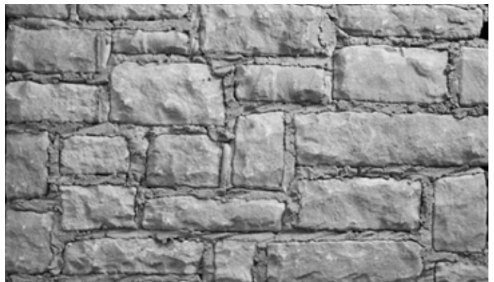
To avoid excessive cutting, lay full units the length of the wall, chasing the cut to a corner or an opening. When cutting or splitting is required, remember to turn the cut edge into the wall and leave the textured ends exposed.
