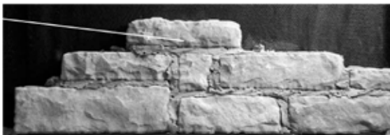
Overlap head joints at least 2" and try not to exceed 3 courses of a vertical joint.
